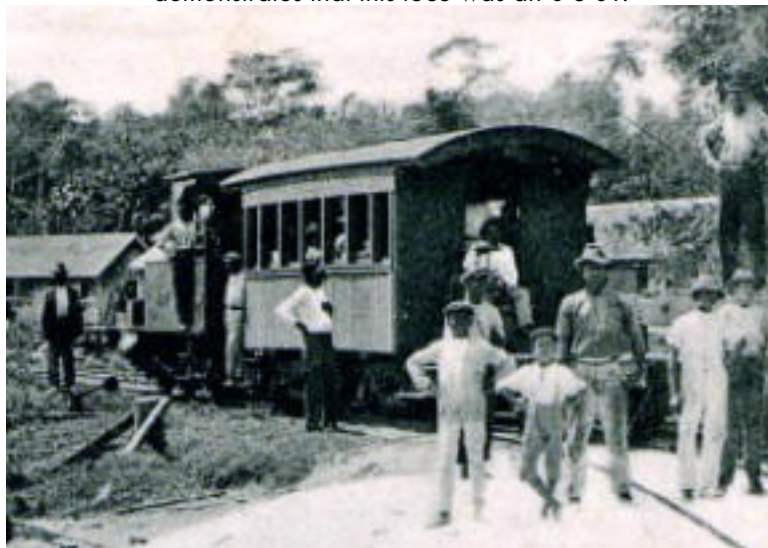
This might well show the same type of loco as was seen above, but if so it looks as the the cab upper backplate has been removed.
