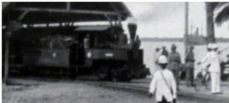
Two images showing Decauville 0-4-0TTs at St. Laurent in the 1920s. As published in Baldwin Locomotives at the time [8]. The tender also appears to bear a Decauville plate.
