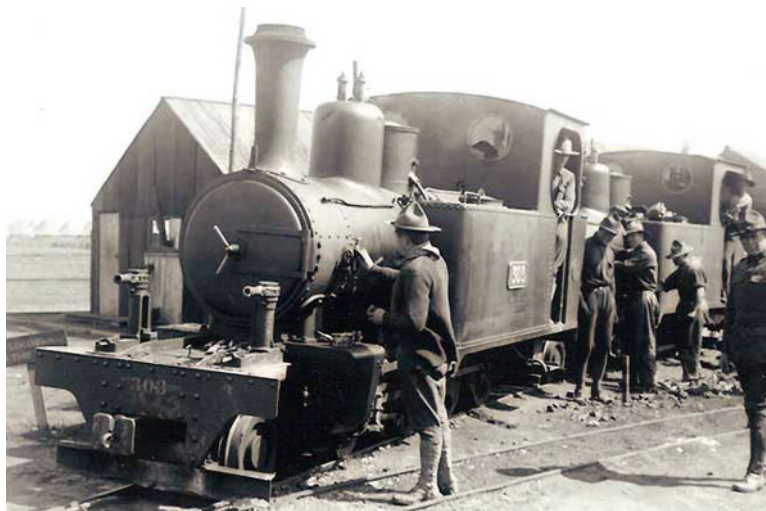
Photo shows similar locos in WD service during WW1.
